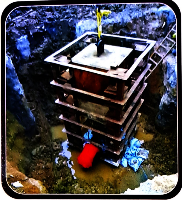
“Pile Load Test”
