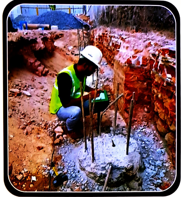
“Pile Integrity Test”
