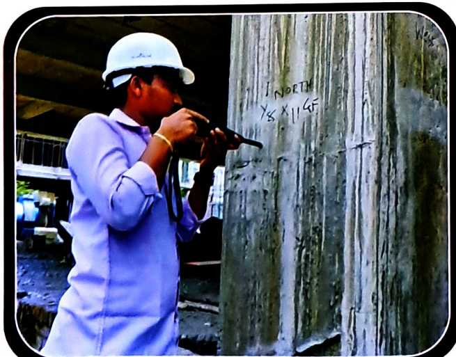
“Rebound Hammer Test”
